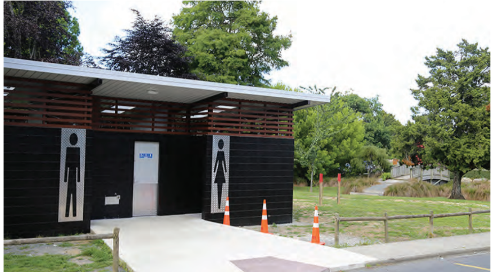
PIOPIO PUBLIC TOILETS AT KARA PARK
