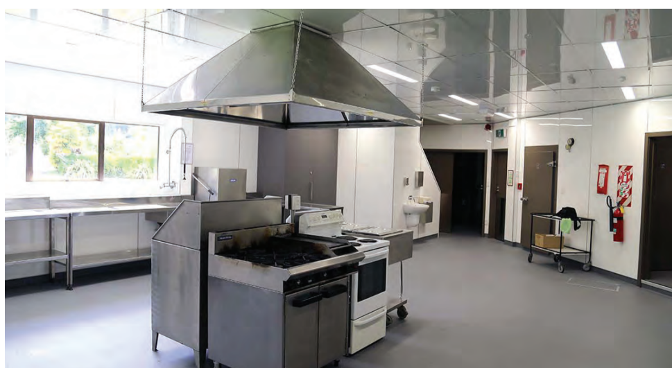
KITCHEN RENEWAL PROJECT AT LES MUNRO CENTRE
