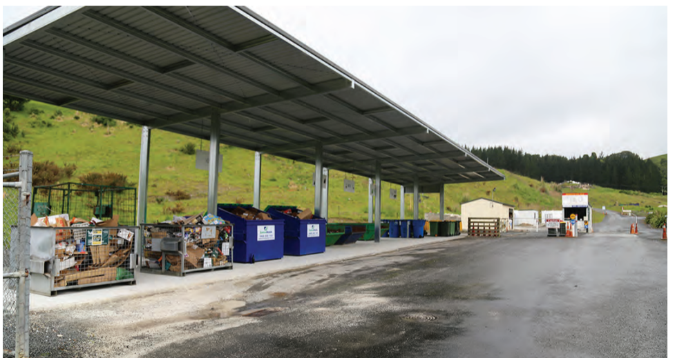
NEW ROOF COVERING THE RECYCLING AREA
