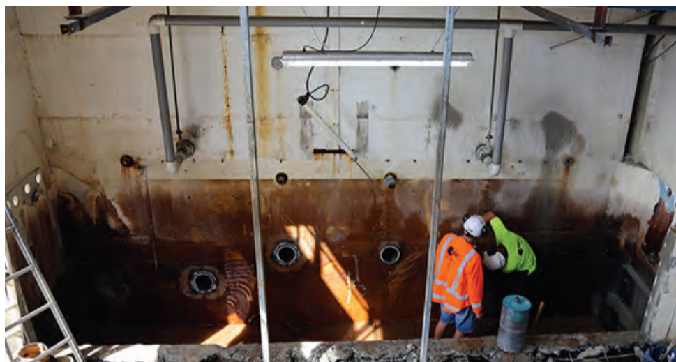
PIPE WORK UNDERWAY AT THE PLANT
